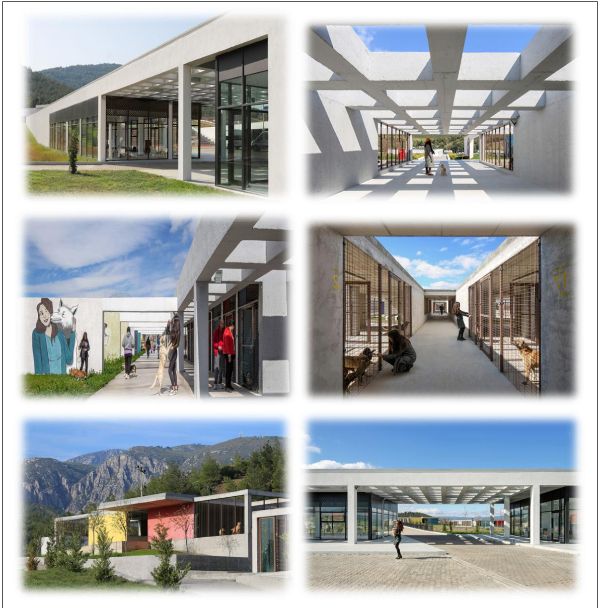
Figure 13.15: Images show the interior/extension zones (source: Search. ArchDaily - Pako Street Animal website)
