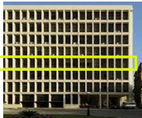
Figure 3. A real-life image of the building's façade is provided, with the third floor highlighted as the focused floor plan for the investigation
