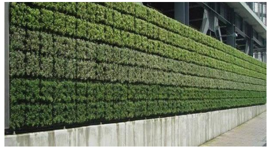
Figure 7. An example of green wall cladding is provided, showcasing its application as a natural sound-absorbing material for façades
