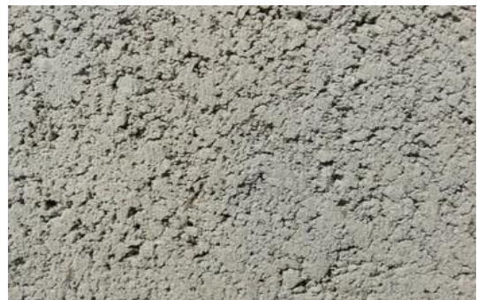
Figure 8. An example of concrete tiles with wide pores is provided, showcasing their application as a sound-absorbing material for façades
