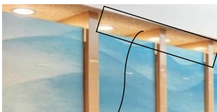
The Bathroom- Wood wool acoustic panels
