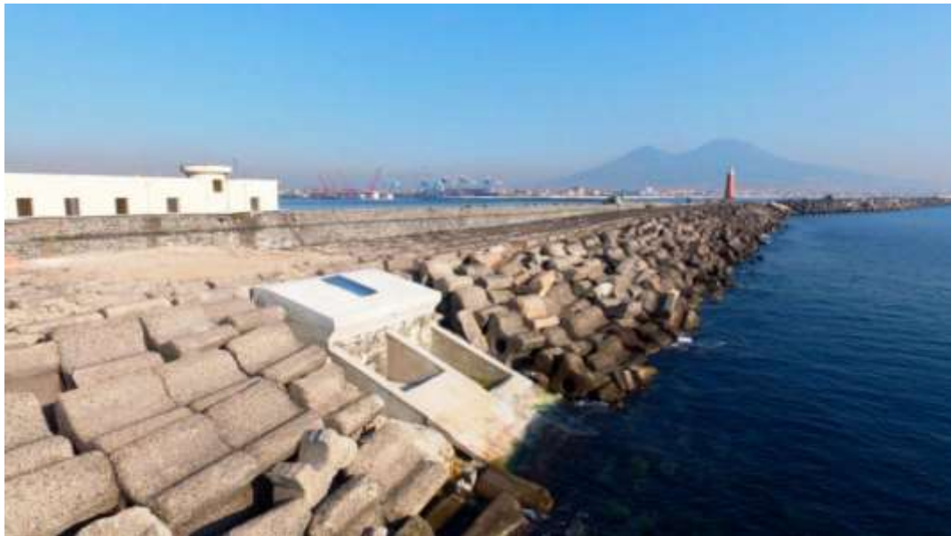
Figure 2. OBREC implementation in Port of Naples [101].
