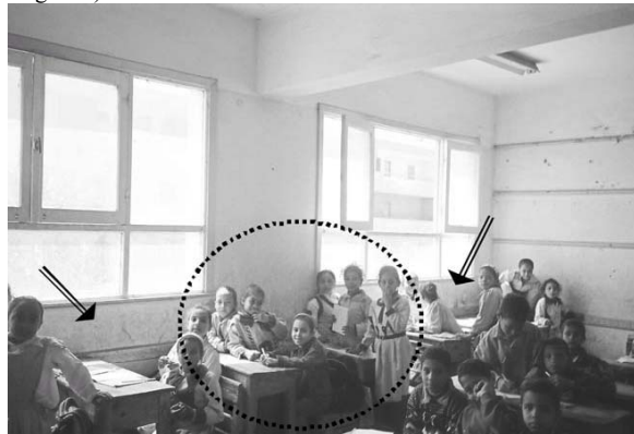
Figure 8: Directed solar radiation falling on the children, after Gado et. al. (Gado et al. 2005)
