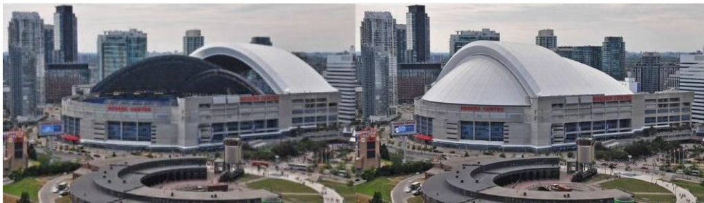
Fig 6: Right, Rogers Center in closed state. Left, half open state(18).
