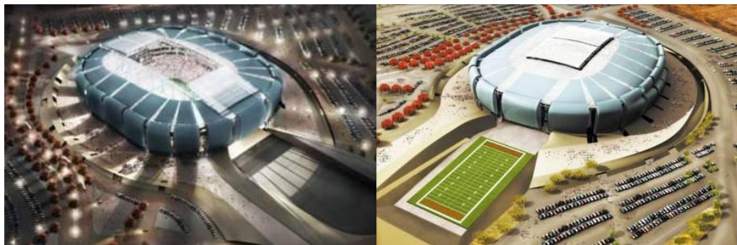
Fig. 8: University of Phoenix stadium: left, at day (closed), right: at night (Open)(1).
