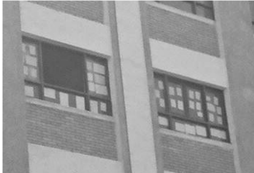
Figure 7: Windows covered and painted by the occupants after Gado and Mohamed (Gado et al. 2005)
