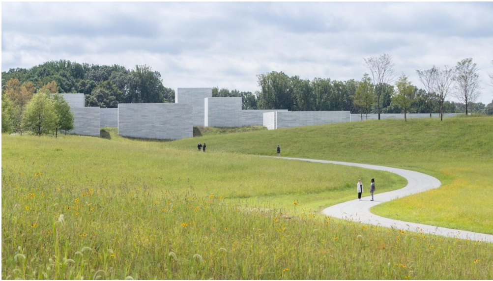
FIGURE 2-18 EXTERIOR OF THE NEW GLENSTONE MUSEUM
